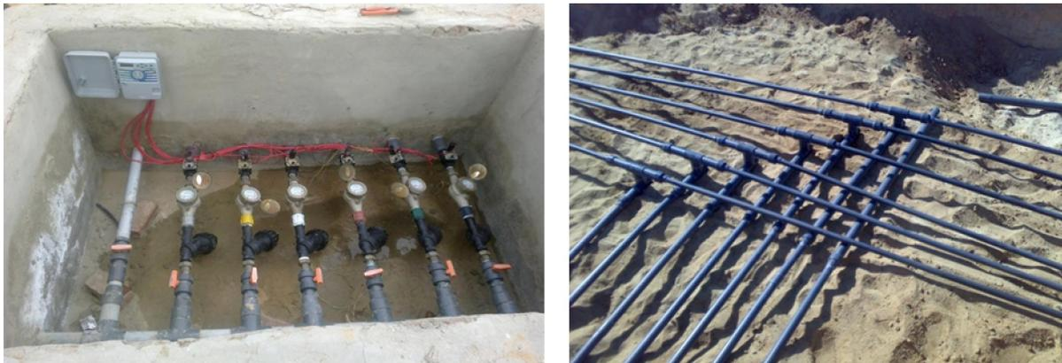
Fig. (2) Irrigation network system (valve box, flow meters and controller) (installation pipes).
