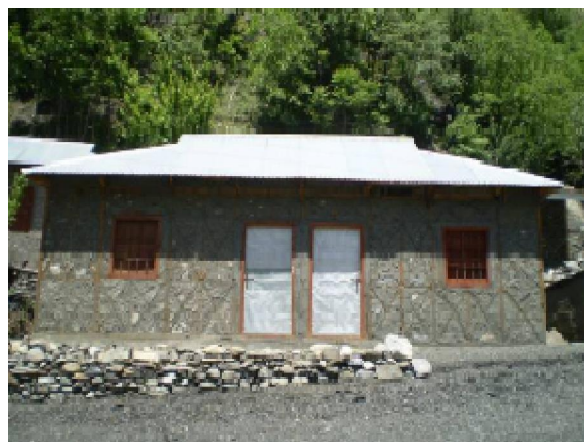
Figure 5(b) Dhajji Structures with dry stone infill in Union Council Pattan Kalan, Abbottabad.
