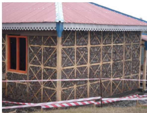
Figure 5(a) Dhajji Structures with mud masonry infill in Union Council Pashto, Battagram
