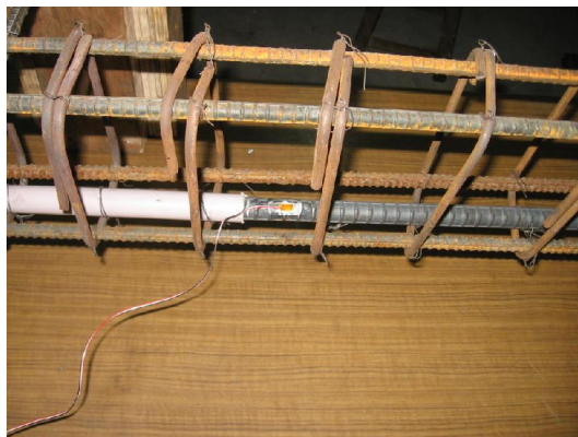
Figure 4. Tied steel with PVC pipe
