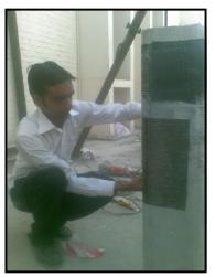
Fig.7 CFRP wrapping on concrete column
