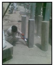
Fig.5 Preparation of columns for confinement of CFRP wrap
