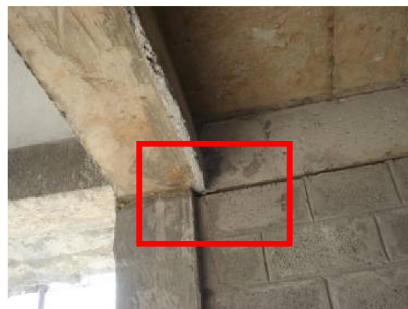
Figure 18: Offset of beam
