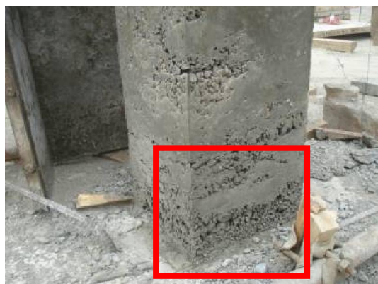
Figure 8: Excessive honey combing in structural column
