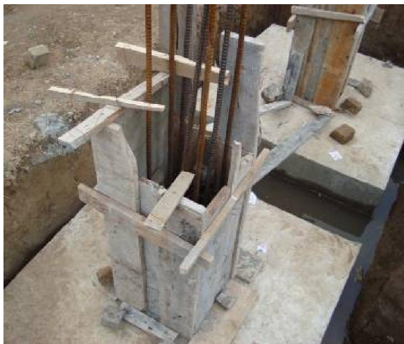
Figure 4: Poor form work and improper concrete cover
