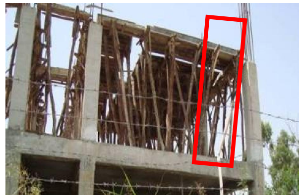
Figure 14: View of column out of plumb
