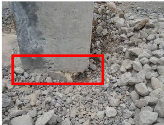
Figure 21: shows a practical example of column rotation in column axis.
