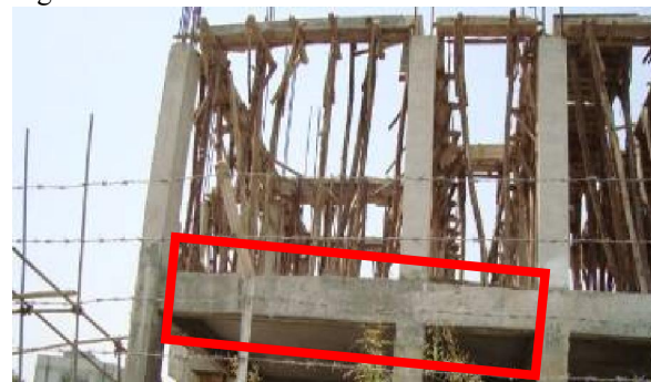
Figure 19: Offset of Beam
