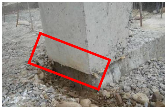
Figure 17: Offset of column
