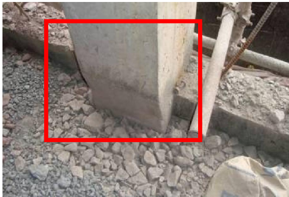
Figure 11: Varying column cross section
