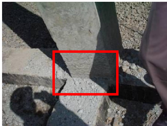
Figure 16: Column off set view
