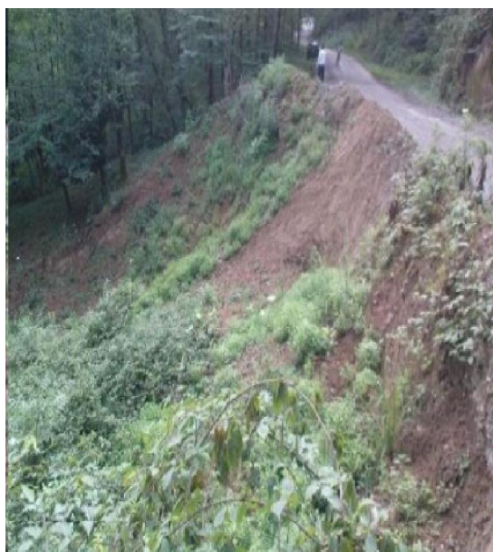
Fig. 5: (a) and (b) Images from new landslide under the communication road between Sharghelt and Aalam-kola - landslide 2.
