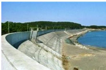
Figure (3): massive concrete wall along the coast
