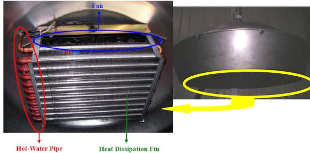
Figure 3. View of Poultry-heater structure
