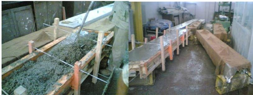
**Fig. 5: Preparation and curing of composite decks**
