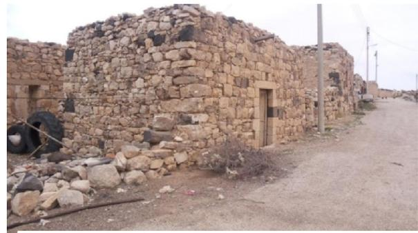
Figure 4 mixer between white lime stone and black basalt in construction, The researcher, 2014
