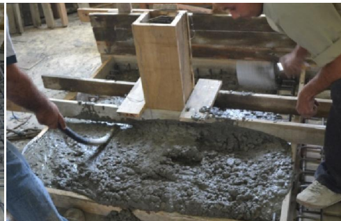
Figure (4): pouring concrete in slabs
