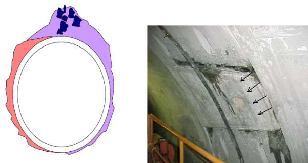
Figure 19. Key segment is pushed out by excessive grouting pressure [11]
