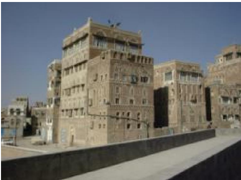
Figure 5: all the building well oriented to the sun and plastered from inside by sand, adobe and scoria (crushed volcanic rock) they are good insulation materials keep the heat inside and make the stone wall very suitable thermal mass . (21)
