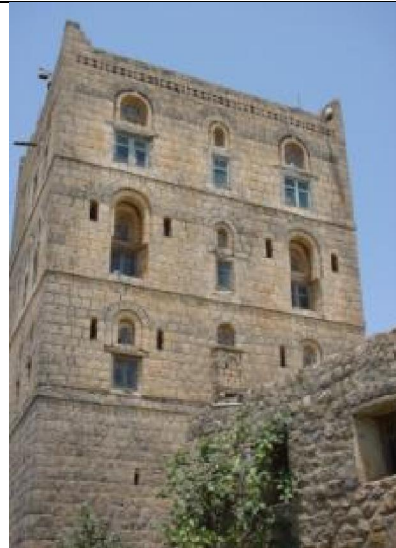
Figure 19: the lower floor of the building solid thick walls with very small opening for ventilation as natural pantries and root cellars to help keep produce and other provisions fresh. (21)
