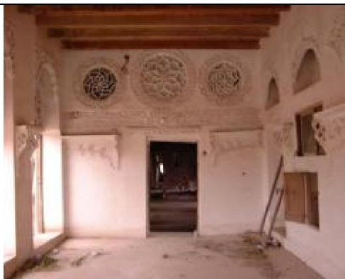
Figure 11: minim use of wood only for ceiling and walls support elements decoration from stone to save forests. (21)
