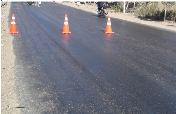
(b) HMA Rutting –Section 7
