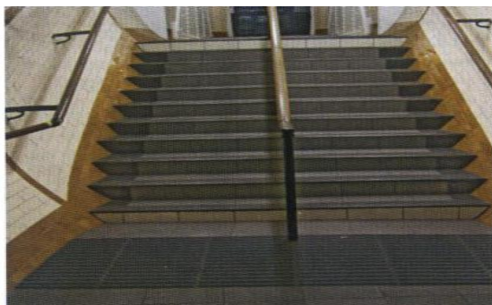
Using grooved touching surfaces on top and down the internal stairs
