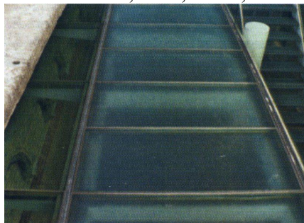
Sandblasted glass supplies enough friction for flooring.
